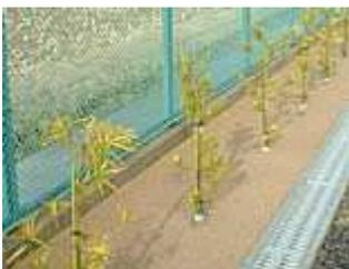
Are you having a problem with weeds that grow with out limitation? The simple execution of "Grass Feud" can confine weeds with a compressed strength of more than 12N/mm<sup>2</sup>, while there is permeability.
